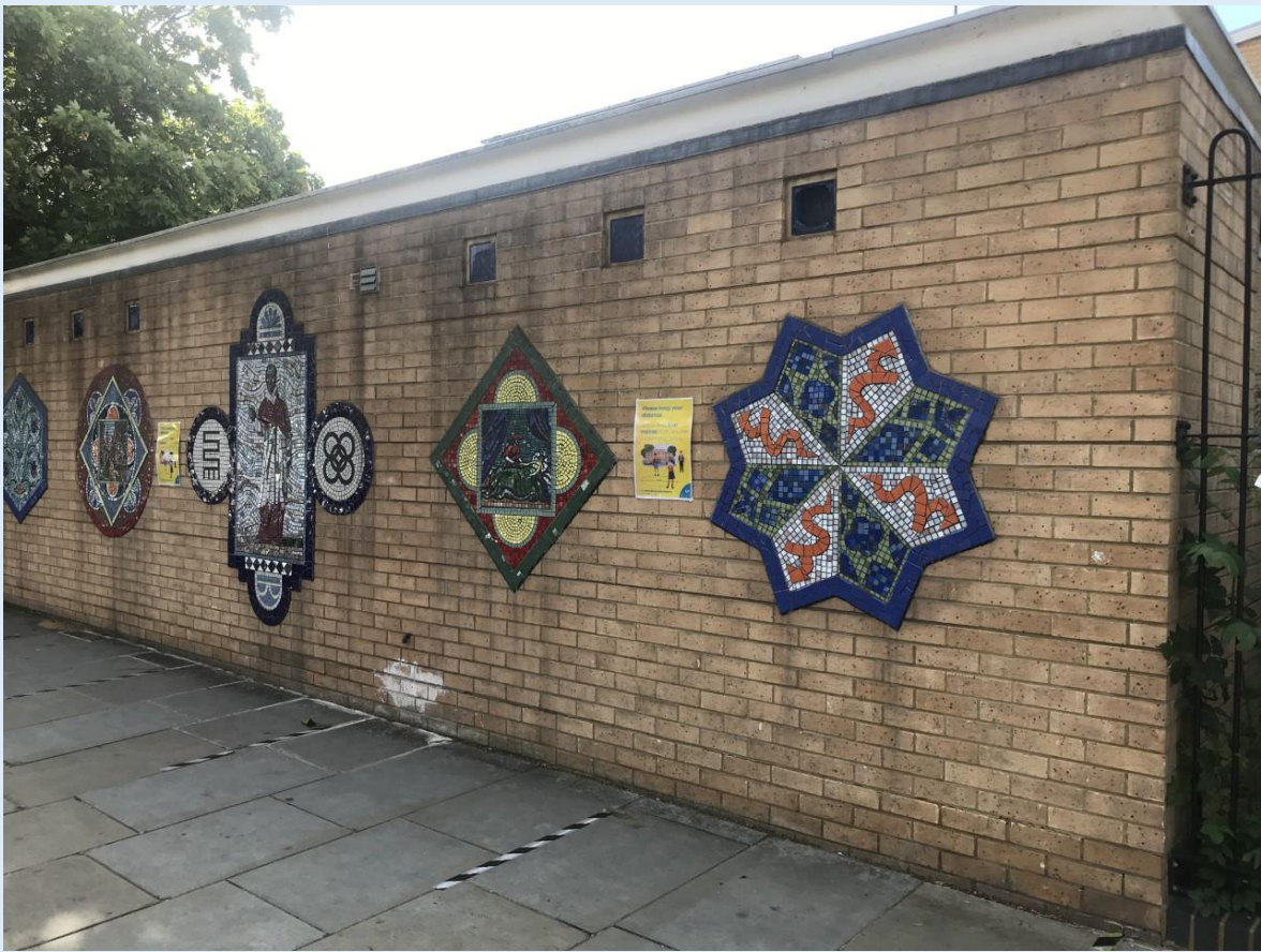
This is what St Charles RC Primary School looks like from the outside.
